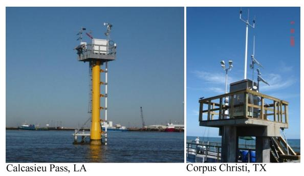
**Figure 3.3**. NOAA tide station installations at (left) Calcasieu Pass, LA and (right) Corpus Christi, TX hardened to withstand major storm surge for continuous long-term operation.
