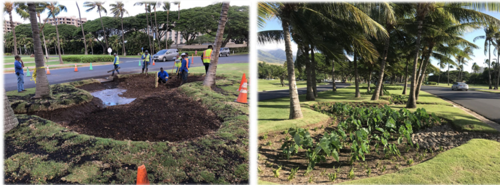
Figure 2-34. Constructing (left) and finished (right) bioretention area in West Maui. Source: West Maui Ridge to Reefs
