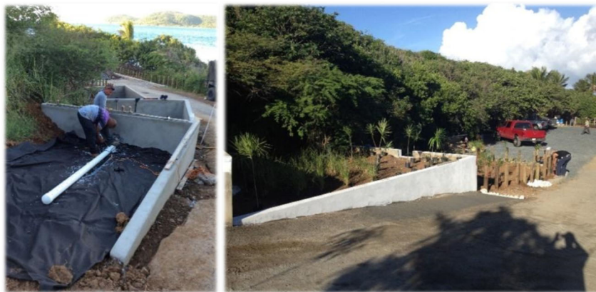
Figure 2-39. Building constructed wetland (left) and finished wetland (right). Source: Protectores de Cuencas
