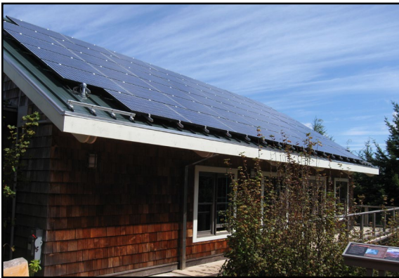
Figure 6.2: Solar panels that are mounted to the roof of the Interpretive Center auditorium.
